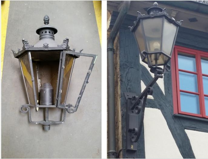
*Before the retrofit: Desolate condition of the existing luminaire body*
