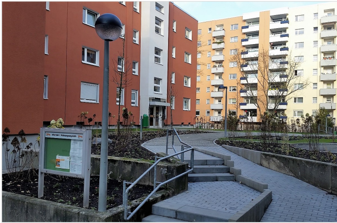
Before Retrofit: Outdated ball light with HQL bulb, unsightly and with high consumption
