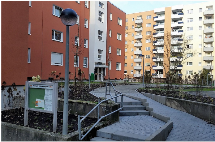
Before Retrofit: Outdated ball light with HQL bulb, unsightly and with high consumption
