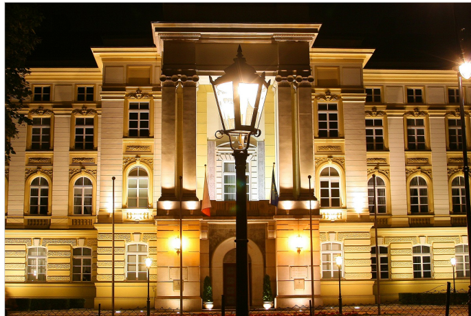
New light for the Warsaw Parliament building
